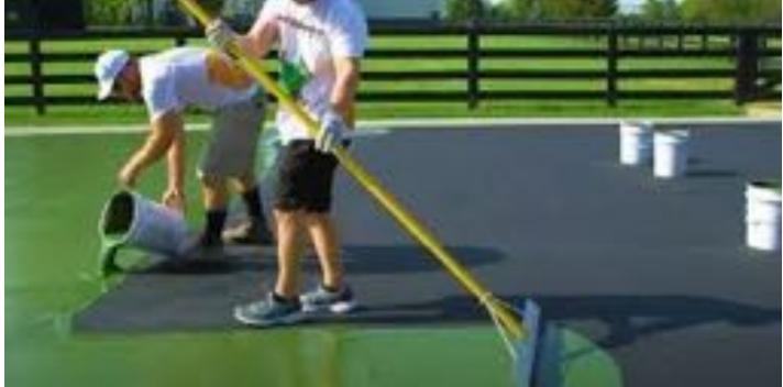
Asphalt courts are made by installing a layer of asphalt on top of a cushion of gravel, then applying an acrylic coating generally over a fiberglass inter layer. These courts are not as durable from a life cycle perspective, especially when installed over this type of soil.
