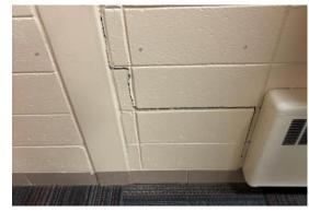
Cracks due to settling of foundation
