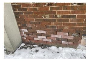
Deterioration of masonry at North facade
