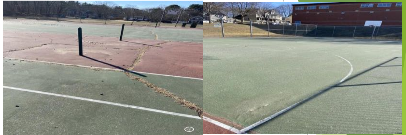
Existing conditions at Barrows
